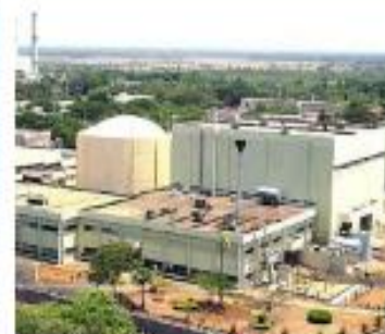
FBTR, 13 MW(e) India, 1985
