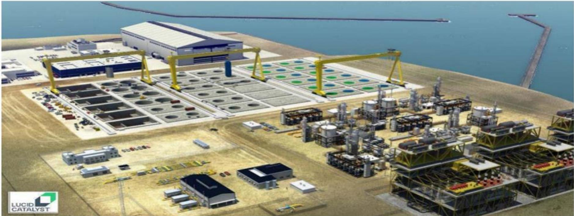
Figure A1.1 – Conceptual illustration with modular manufacturing and assembly building at rear, hydrogen gigafactory under construction beneath the yellow cranes, adjacent hydrogen manufacturing plant and liquid synthetic fuel manufacturing plant in the foreground
