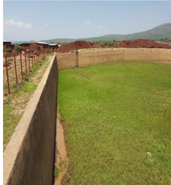
An empty artificial water catchment basin in Southern Ethiopia
