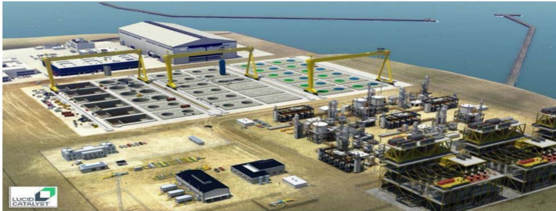
Figure A1.1 – Conceptual illustration with modular manufacturing and assembly building at rear, hydrogen gigafactory under construction beneath the yellow cranes, adjacent hydrogen manufacturing plant and liquid synthetic fuel manufacturing plant in the foreground
