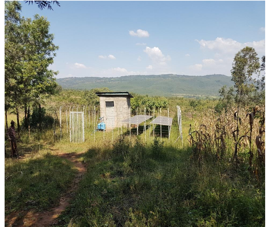
Drip irrigation system powered by solar energy installed in Ampo Koysha, Wolayta, Southern Ethiopia
