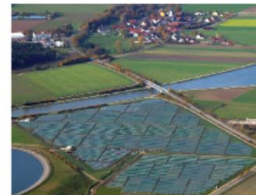
Figure 6.7. A solar photovoltaic farm: the 6.3 MW (peak) Solarpark in Mühlhausen, Bavaria. Its average power per unit land area is expected to be about 5 W/m². Photo by SunPower.
